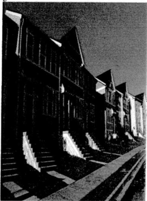
Completed units at Henson Ridge.
