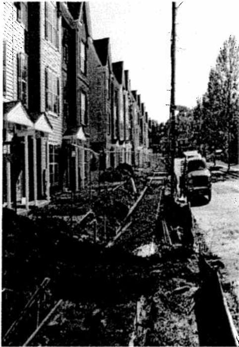
Construction in progress at Capitol Gateway (formerly East Capitol).
