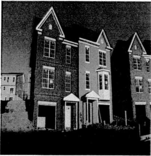
Partially completed single-family homes at Capitol Gateway.
