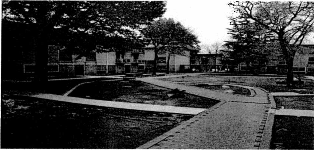
Sidewalk renovation in progress at Kentucky Courts. Renovation was funded by Bond funds.
