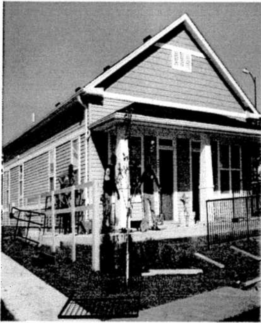
A nearly completed UFAS unit at Henson Ridge.
