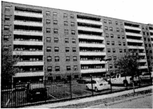
Renovated balconies at Greenleaf Senior as part of Bond funded modernization efforts.
