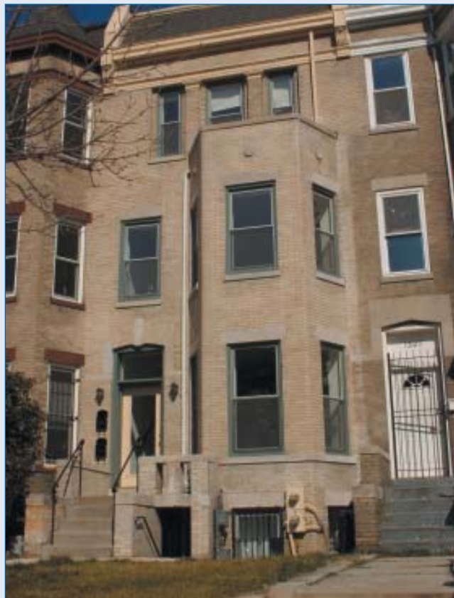
This property, located in Columbia Heights, is one of 78 currently being renovated for homeownership by DCHA and a team of non-profit developers.
